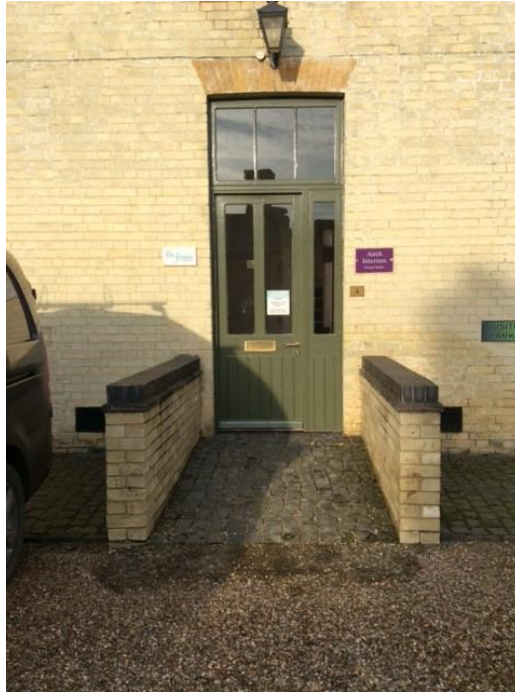
Image of external door leading to toilet 1
